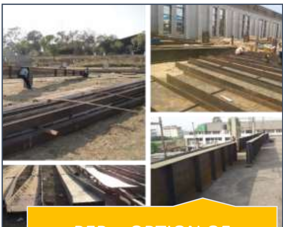
PEB – OPTION OF FABRICATION ON SITE
